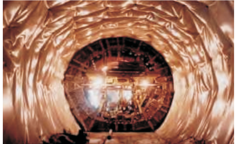
Fixation of the geomembrane by spot welding
