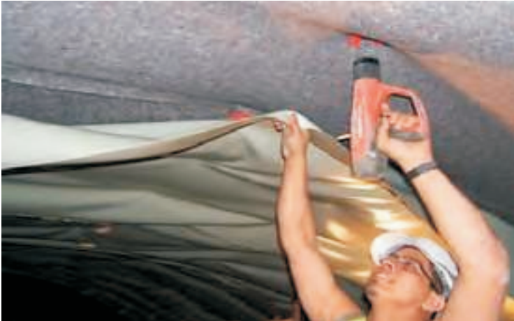
Fixation of the geotextile
