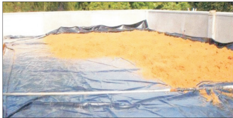
Geomembranes with welded water stops produced in prefabrication
