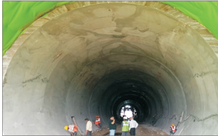
Installation of membrane
